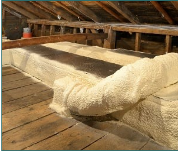
Commercial building duct sealing energy savings and cost analysis
