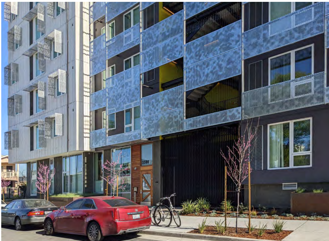
Case Studies of All-Electric Multifamily Residential Buildings
