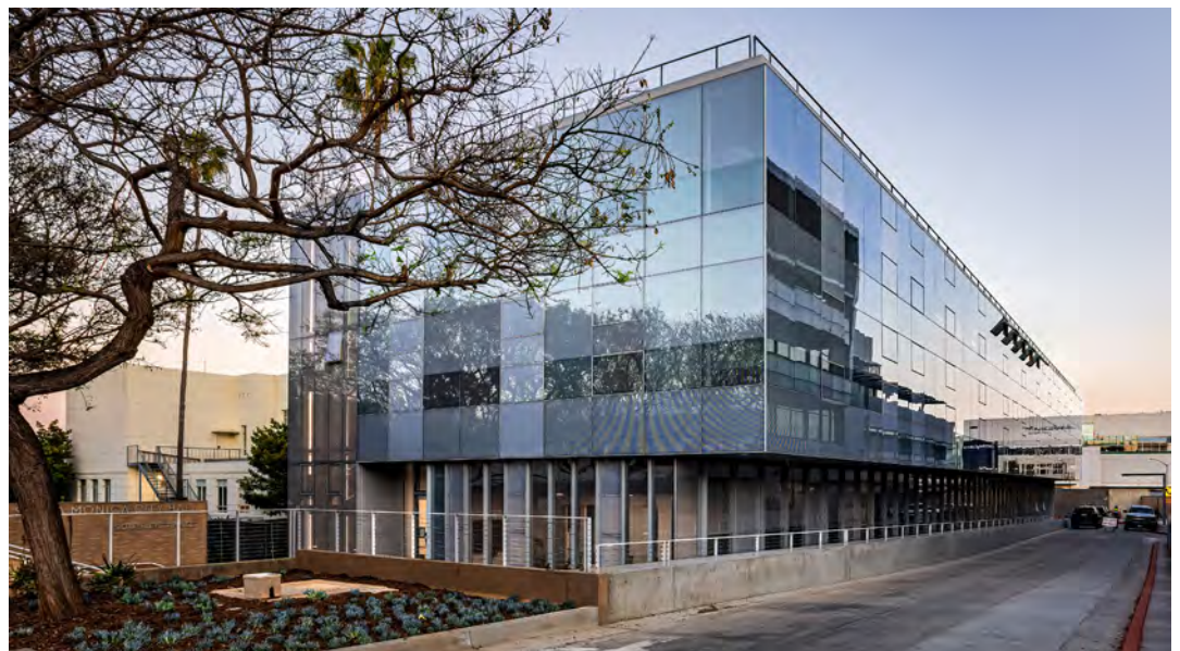
(Right) View of new City Hall East building from the south, with the curtain wall visible on the south and east elevations (Photo: Randall Howard)
