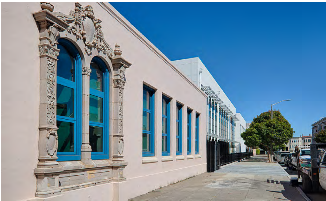
(Left) View along North Point Street, existing historic building at left and new middle school street facade beyond. (Photo: © Technical Imagery Studios)
